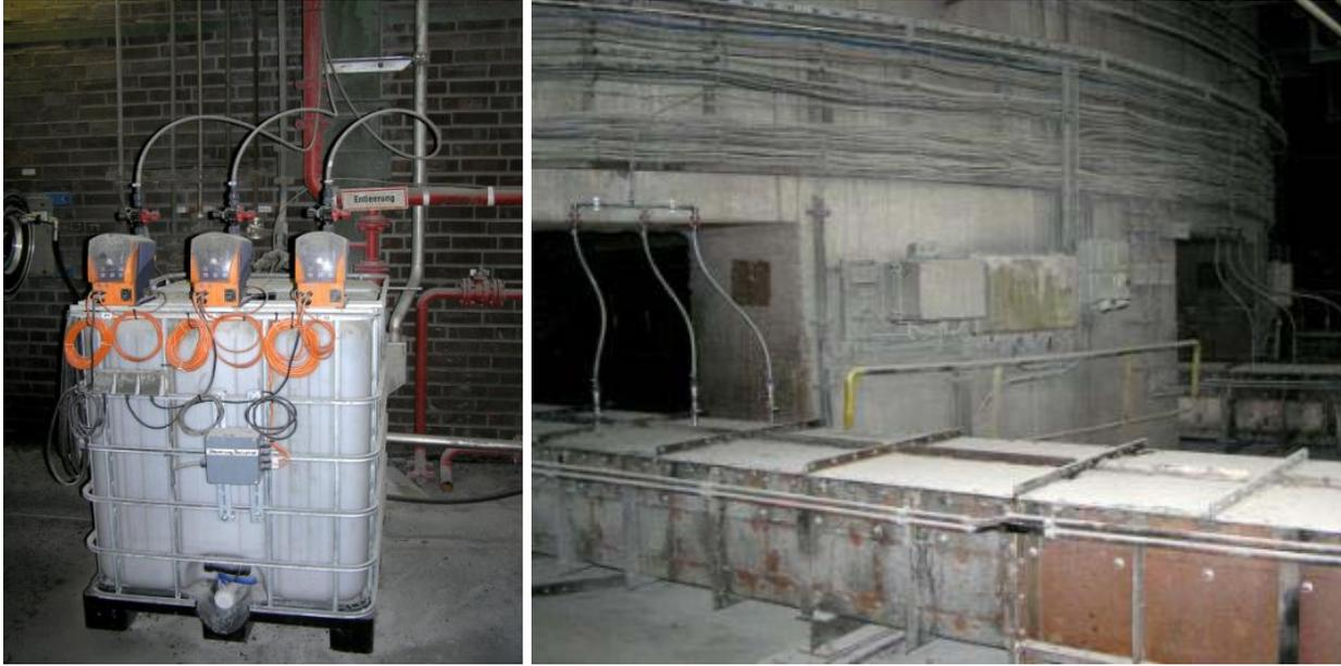
**Figure 4:** CaBr<sub>2</sub> addition from totes to coal feeders underneath the day bunkers
