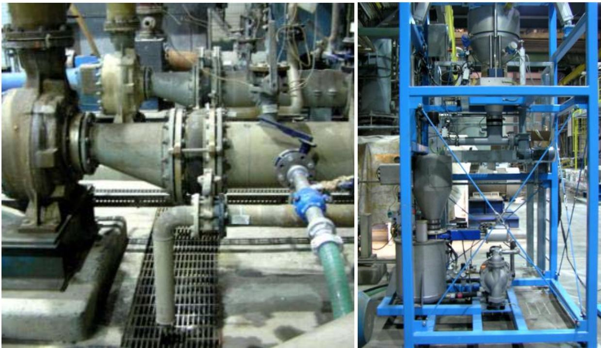
**Figure 5:** PAC dosing station and injection point into the suction side of an absorber recycle pump
